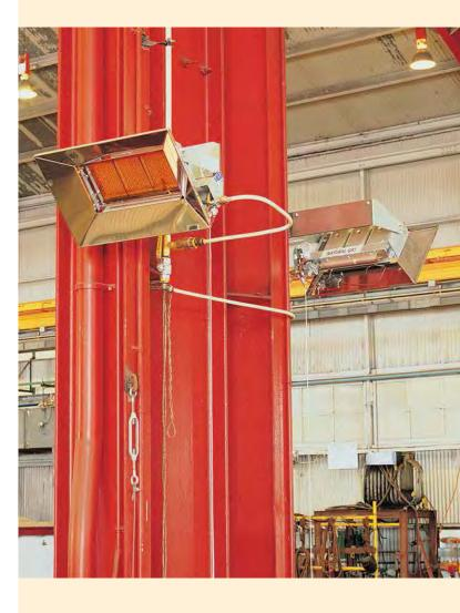
In commercial use this allows selected indoor areas to be heated to comfort level without raising the temperature away from that immediate position. This quality is unique to infra-red heating and can effect great saving in fuel costs. Zone or broad heating is achieved by positioning specified numbers or combinations of heaters at appropriate heights and locations.
